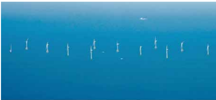
Alpha Ventus Goes Online: At a height of 150 meters (492 feet), each turbine is as tall as Cologne Cathedral and, at 1,000 tons, as heavy as 25 fully loaded semi-trailer trucks. Source: Spiegel online: www.spiegel.de/international
